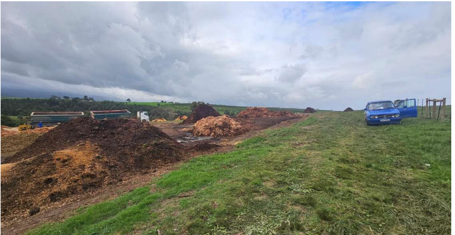
Photo showing the composting site from west in an easterly direction. The site is on the southern side of the DR 1599. The southern boundary of the farm, corresponds with the fence to the right side of the car. The DR 1599 is situated to the left side of the photo, appr 100m 150m from the car. The road divides this portion of Farm 29/227 from the larger portion thereof which is located to the north of the road.
