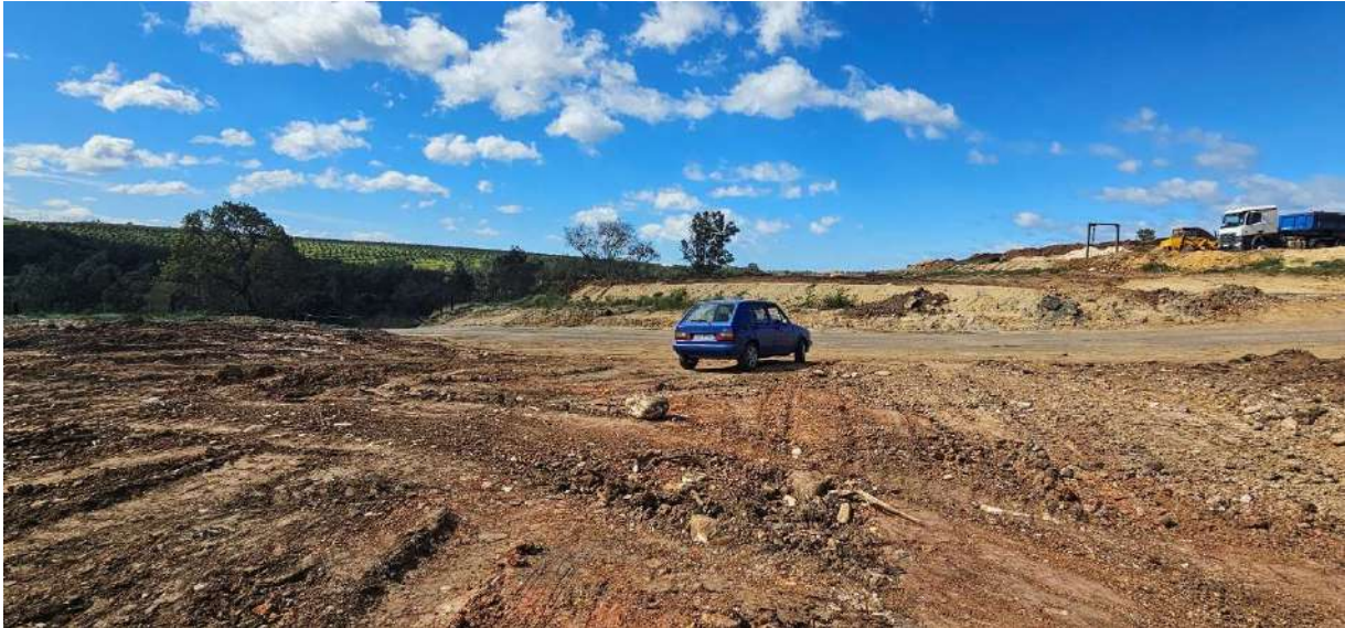
Photo 9 The photo shows the fill platforms that were created to limit run-off from the site.
