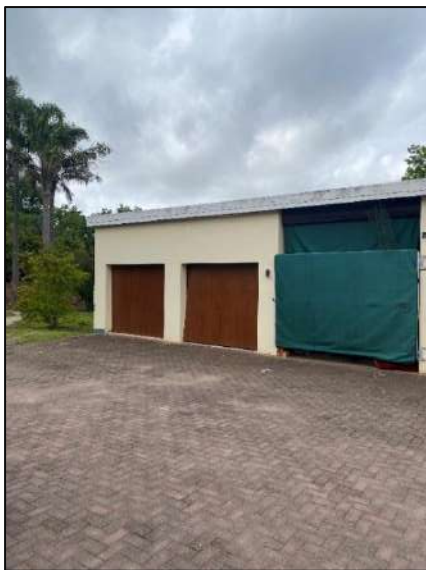
Figure 7: Garage section located southmost of the maids' quarters
