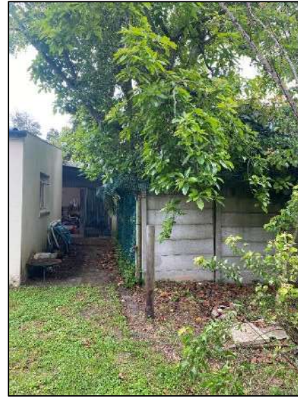
Figure 13: Communal wall between subject erf and abutting erven.
