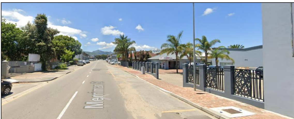
Figure 4: Photo of surrounding developments (taken northwards towards Hibernia Street)
