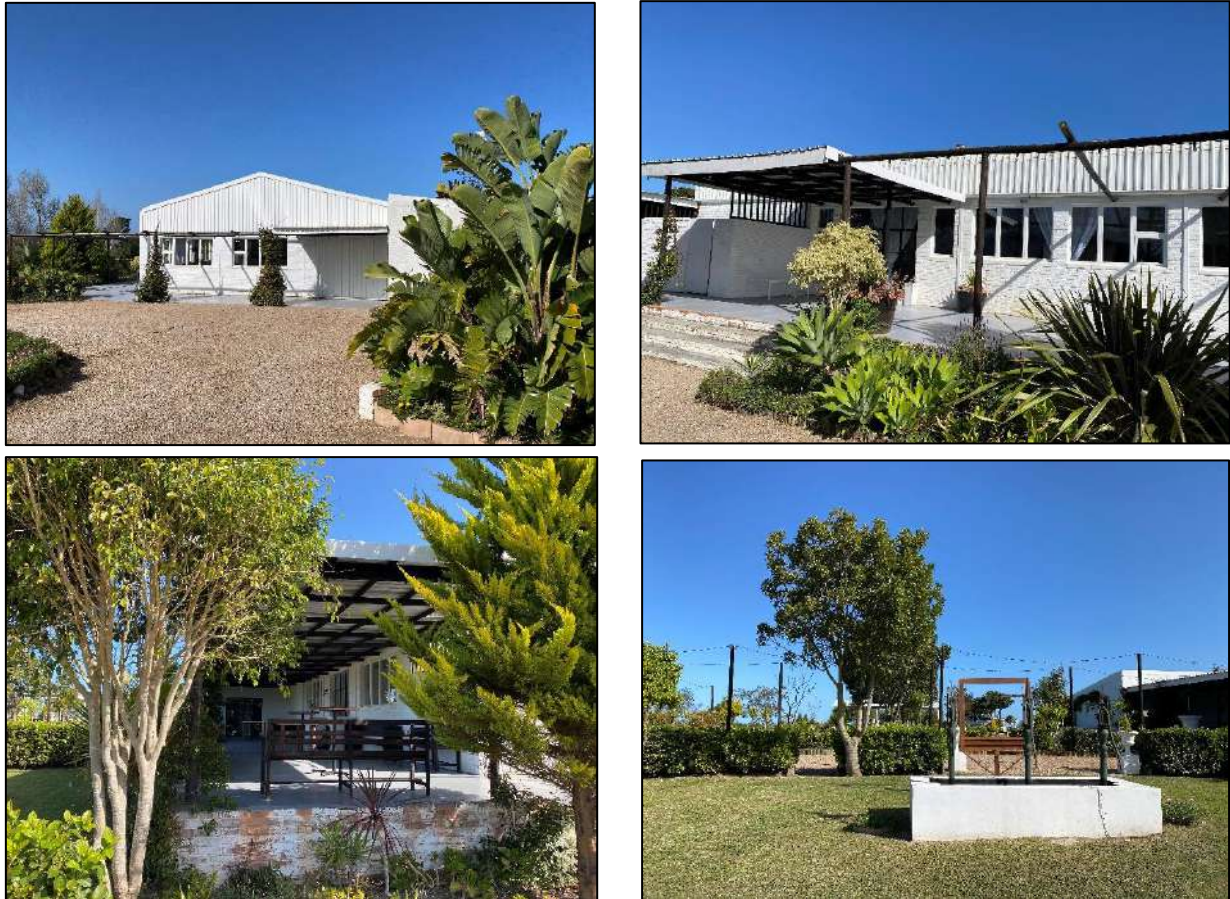
Figure 7: Various photos of the reception hall and surrounds
