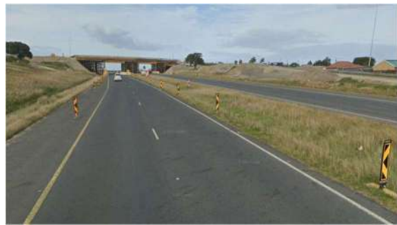
Figure 3.9: Existing National Route 2
