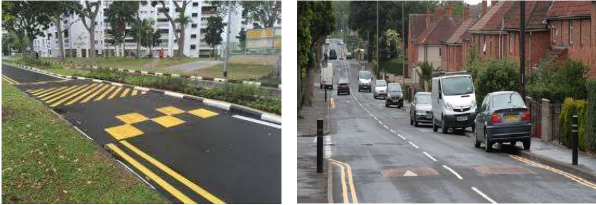
Figure 6.11: Bus friendly speed hump or Speed cushions (Sources: Reinforced concrete road safety: world experience for Cherkasy - 18000.com.ua & Speed Cushions | Traffic Choices - aiding traffic scheme decisions)
