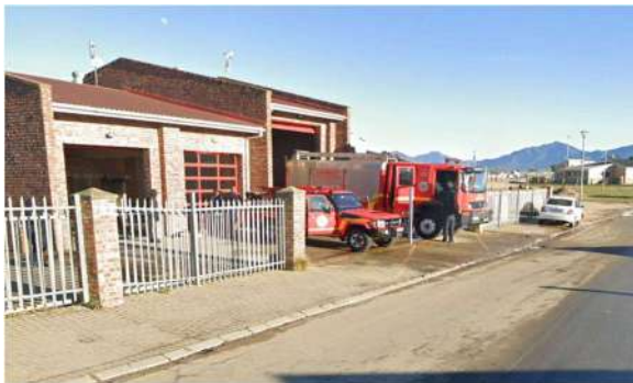
Figure 3.16: Access 5 to Thembalethu Fire Station
