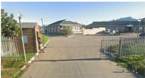
Figure 3.18: Access 7 to Thusong Centre
