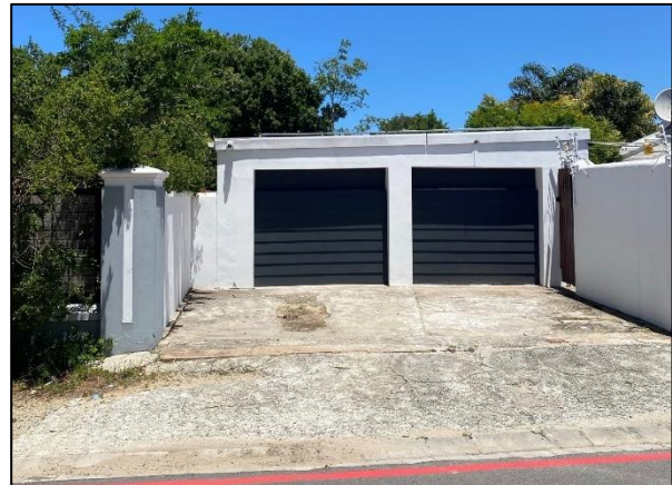
Figure 6: Access to the garage from Drostdy Avenue (to be converted)
