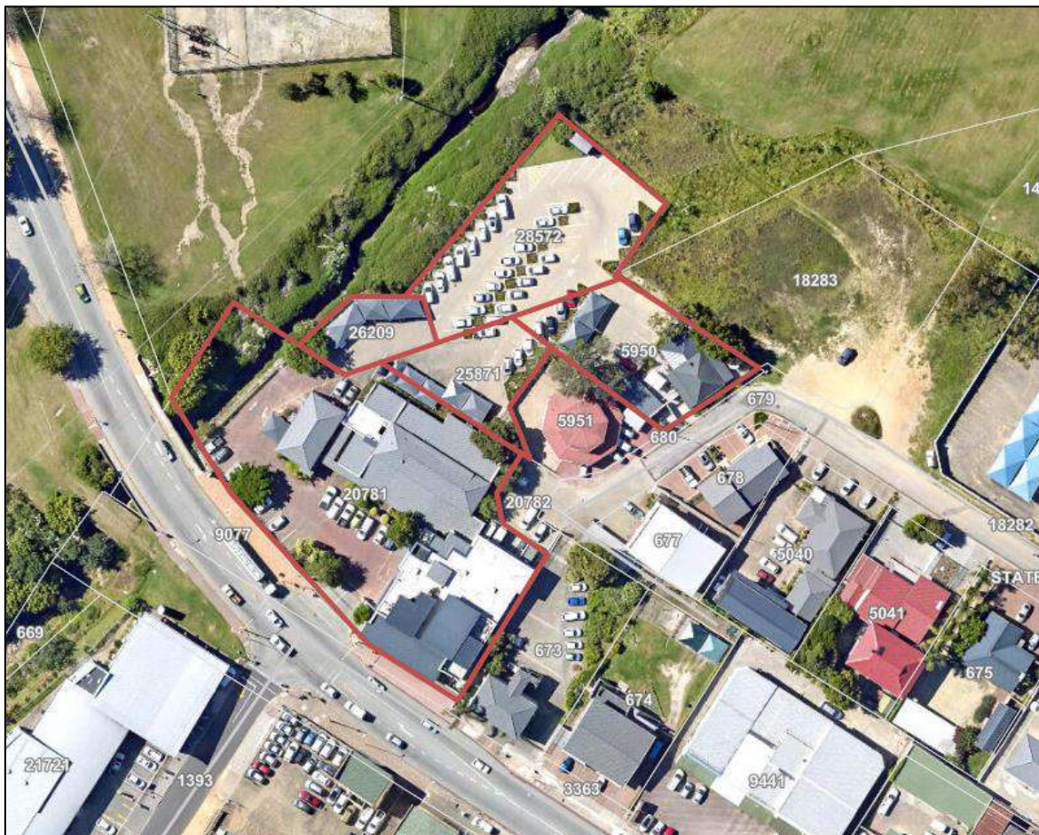
Figure 2: Detailed view of subject property and immediate surrounding land uses
