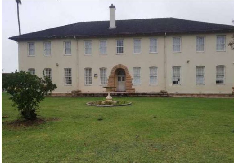
Photo 41(From Die Bult Facebook Page): See the Streetscape Reference Key Map on Page 36 - 'Die Bult' High School Founded 01 December 1912 – Provincial Heritage Site.
