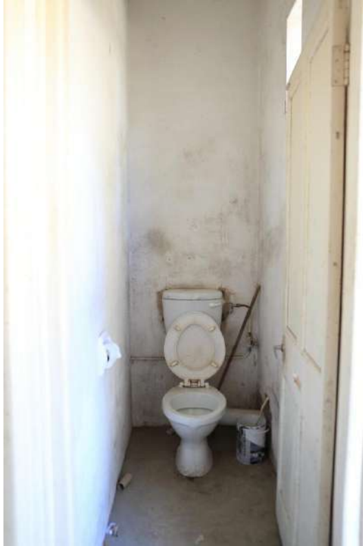
Photo S – WC 2
