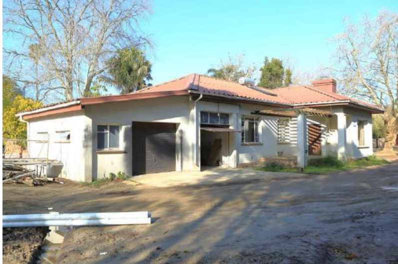
Photo C- The North-Eastern View
