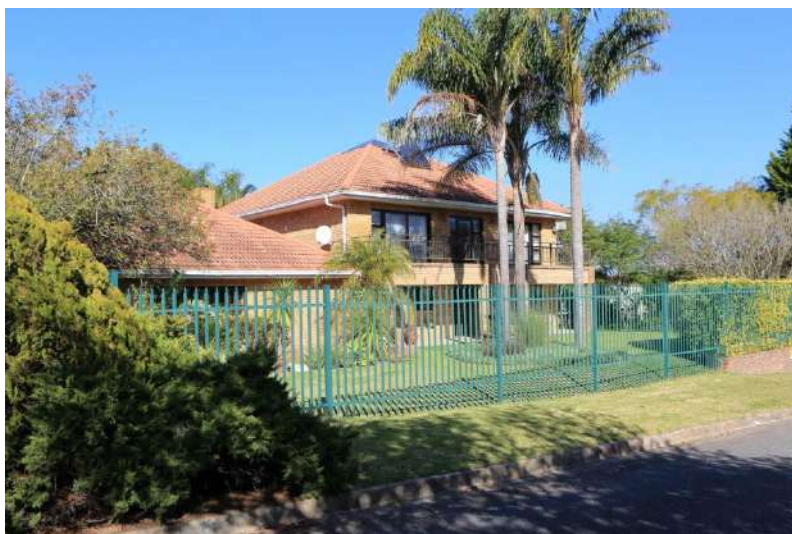
Photo 33 - Looking at ERF 7189
