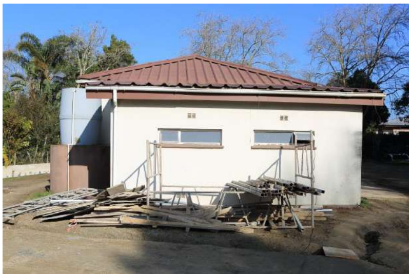
Photo E - Eastern Elevation
