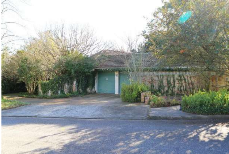
Photo 28 – Looking at ERF 6334
