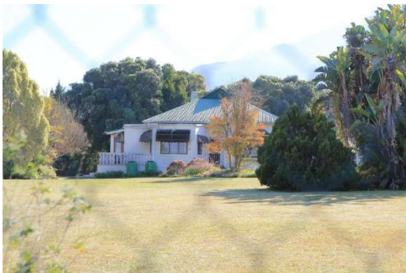
Photo 36- Looking at ERF 7191 (Possibly older than 60 years)
