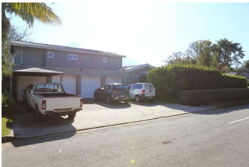
Photo 30 - Looking at ERF 5830
