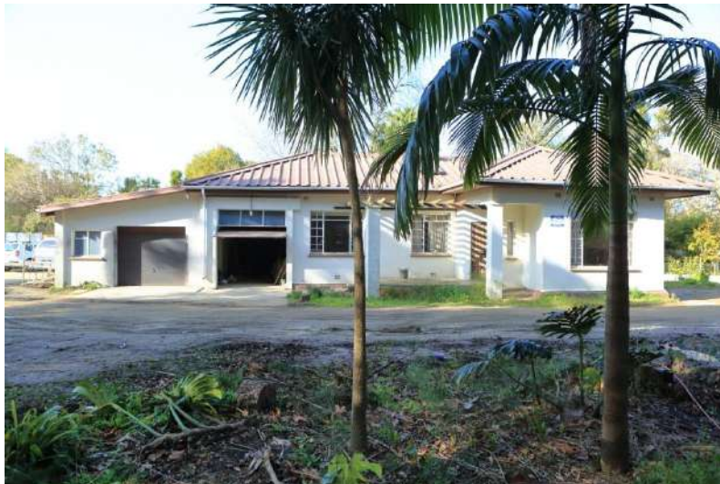
Photo B - The North Elevation.
