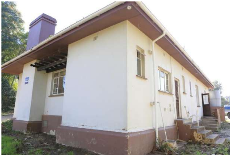
Photo G - The South-Western View
