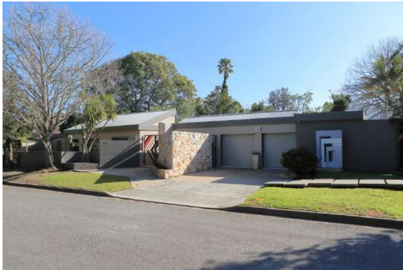
Photo 29 - Looking at ERF 5829
