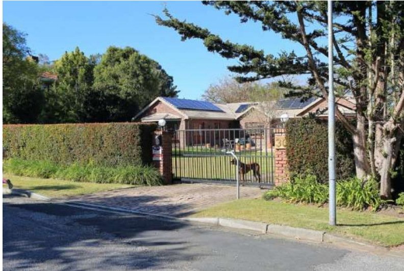
Photo 34 - Looking at ERF 9539
