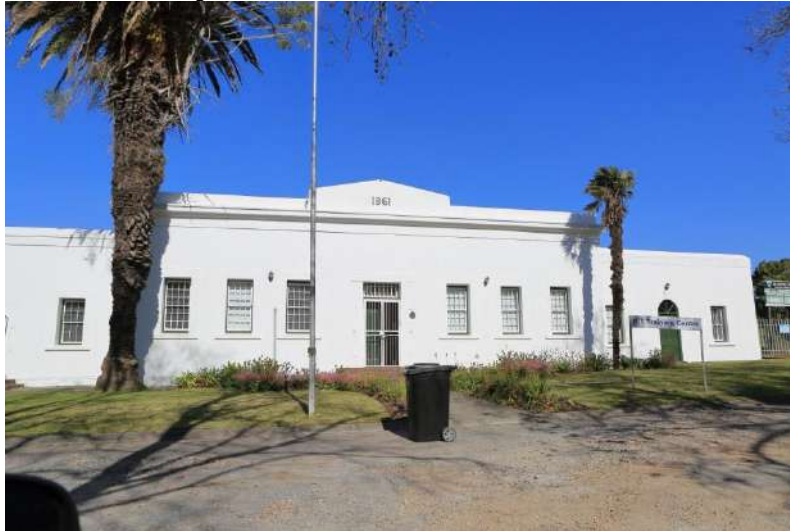
Photo 39: See the Streetscape Reference Key Map on Page 36 - The ICT Training Centre 1861. Provincial Heritage Site.
