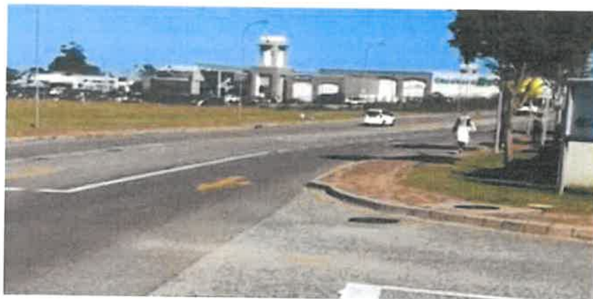
Figure 5: View to the Right: Contractor Access along Park Road
