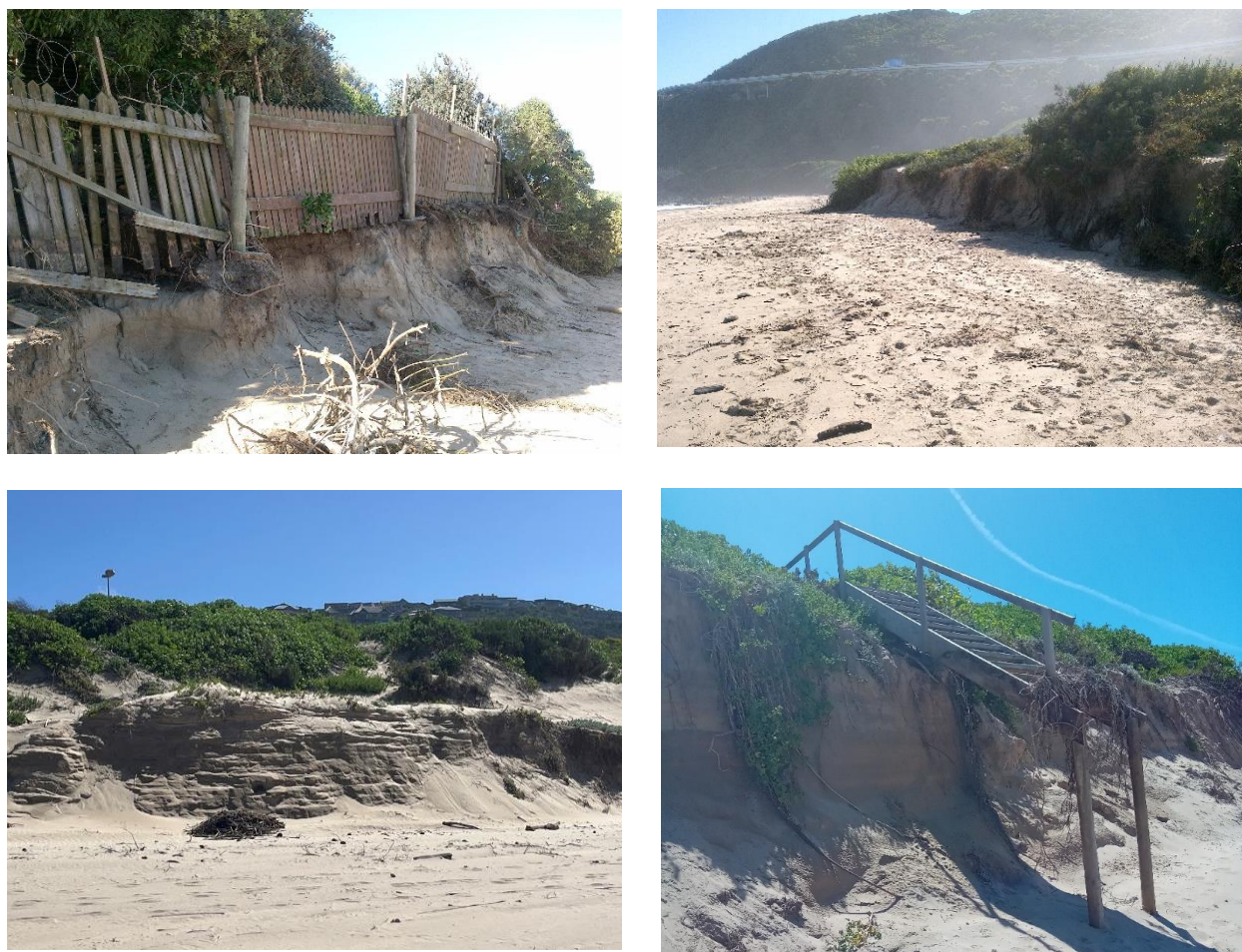
Figure 4. Photographic evidence coastal erosion resulting from the September 2023 storm surge.
