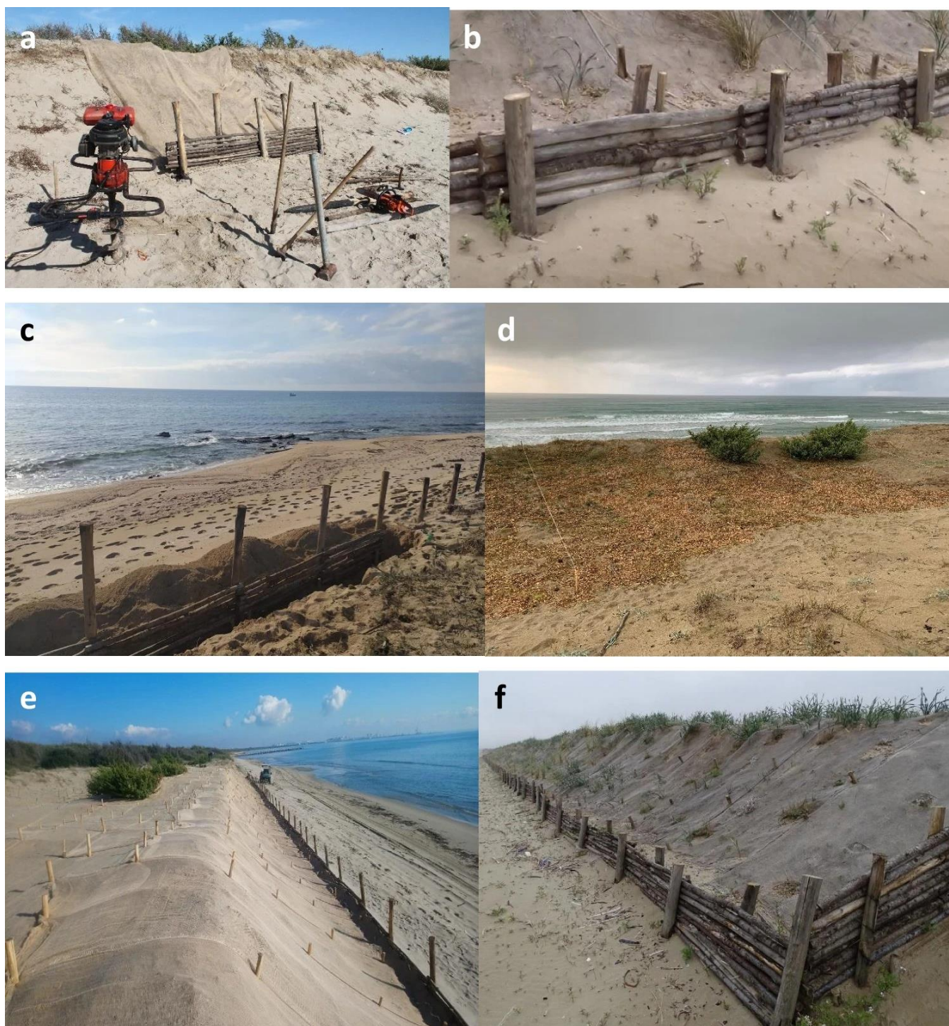
Figure 11. Soil bioengineering technique for coastal dune restoration in the Mediterranean using autochthonous vegetation species. Stages of intervention: (a) pole drilling; (b) wattle; (c) trench excavation; (d) wood chips spreading; e bio-mesh; (f) intervention accomplished 27 .
