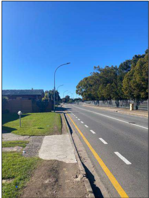
Figure 7: Meyer Street towards the East
