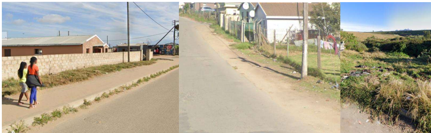
Figure 5-1: Sidewalk conditions along the recreation route
