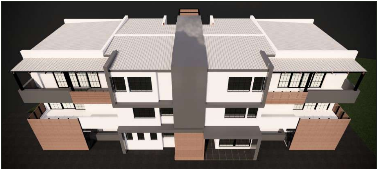
Figure 7: Building back view
