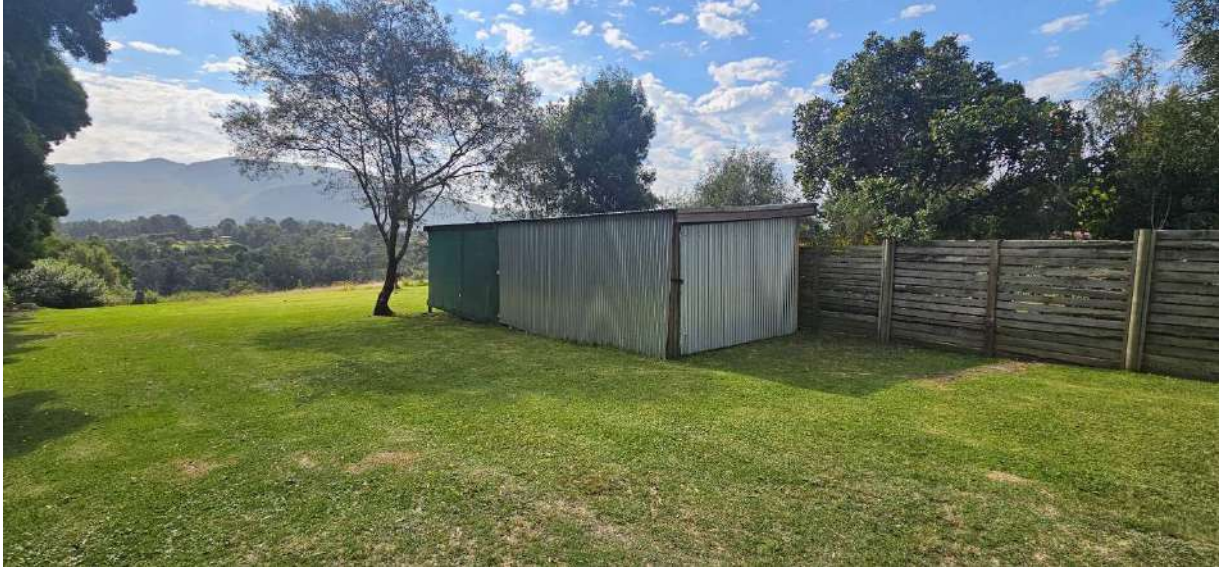
Photo 6 A structure used as carport and shed on the western side of the erf. This structure was erected over the building line by previous owners with slight modifications by current owner and a relaxation is therefore required. The photo was taken in a northerly direction.
