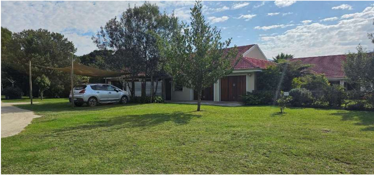
Photo 2 An existing building containing garages and storeroom. The photo was taken in a north-westerly direction
