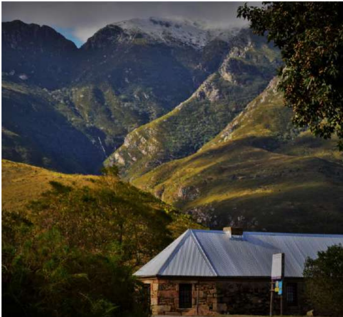
Featured: Old Toll House at Montagu Pass
