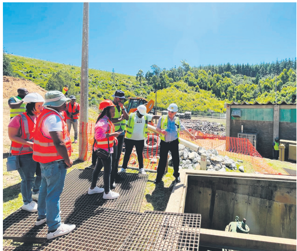
Garden Route Dam Suction Pipework : At pump mains connection chamber – Andre Scheepers, CES Project Manager (BFI) in in the photograph pointing out details to the National Treasury officials.
